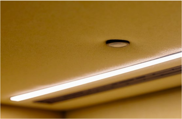
COLOUR TEMPERATURE: 2.700 K ENERGY: 14.4 WATT SENSOR OPERATED: YES MATERIAL: ALUMINIUM LENGTH STRIP: 80CM
