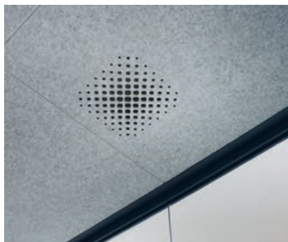
Fresh air is drawn into the room via an invisible sound absorber integrated in the acoustic ceiling
